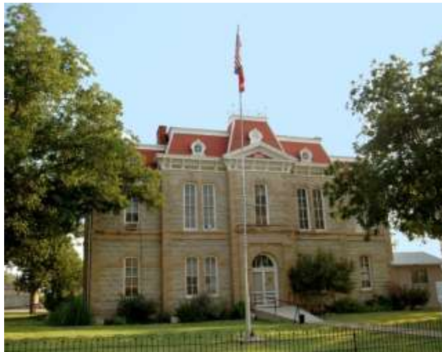
Concho County Courthouse – Paint Rock, Texas
