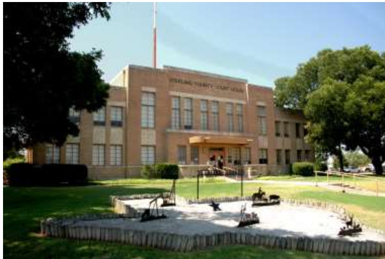
Sterling County Courthouse - Sterling City, Texas
